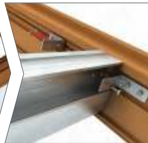
Fix rafters to ring beam
