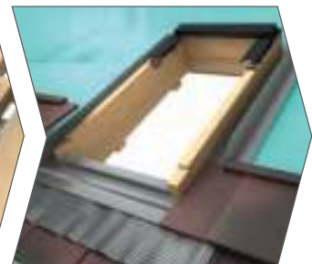
Install roof window
