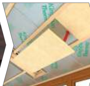
Install insulation between batten
