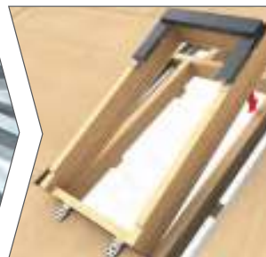
Install roof window frame
